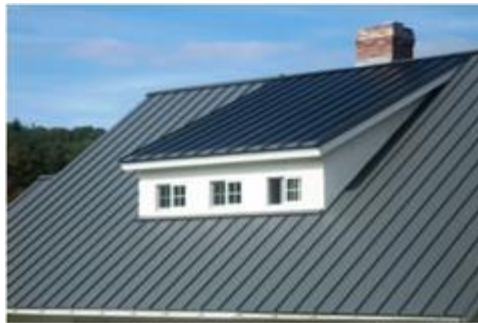
Figure 95-1: Building-Integrated Solar Energy System
