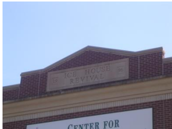
Masonry Parapet Sign
