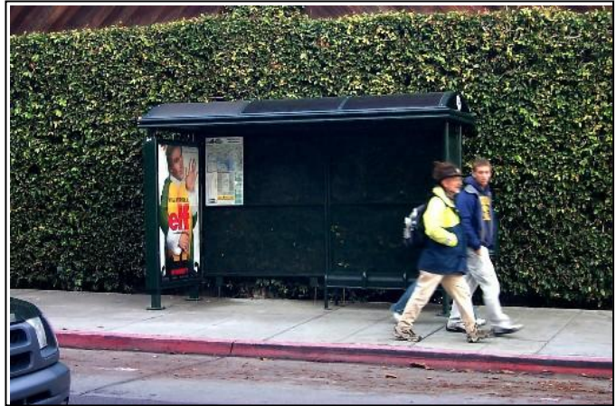
• Figure 26 Bus shelters are needed in the 6th Street Neighborhood.
